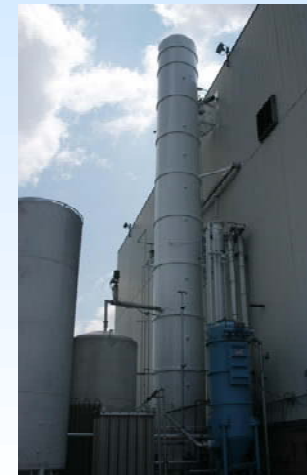
ONE OF SEVERAL ARENCIBIA “COLD BOX” CONDENSERS IN OPERATION
